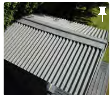
Corrugated roof sheets
